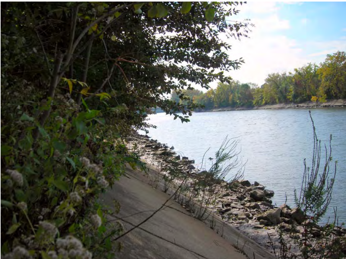
Photo 6. Concrete stabilization wall at RM13.6 (Memorial Park). Wall extends along the entire area sampled.
