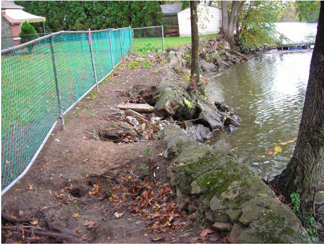
Photo 11. Retaining wall along RM12.3 (Van Winkle Park) crumbling in several places.
