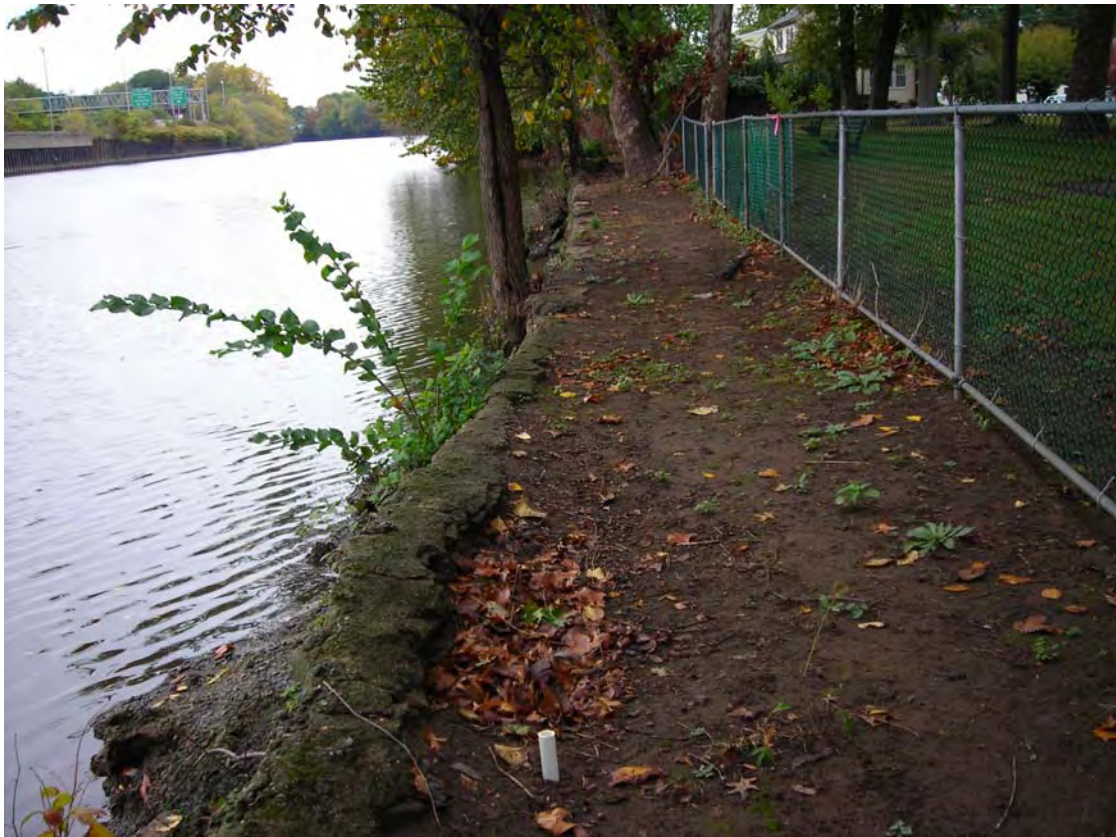
Photo 12. Shows lack of riparian vegetation at RM12.3 (Van Winkle Park).
